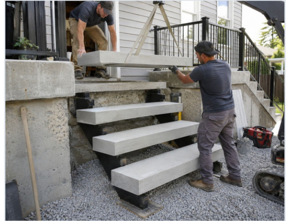
Example: precast stair components during installation.
